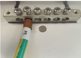
▲ Figure 4.10 Grounding Terminal on Heat-Sink
